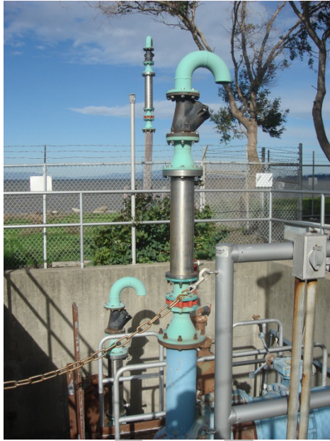
Figure 14-9. Air/Surge Relief Valves at Rodeo Sanitary District's Vault Structure
