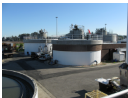
Anaerobic Digesters
