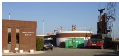
The Pinole/Hercules Water Pollution Control Plant in Pinole
