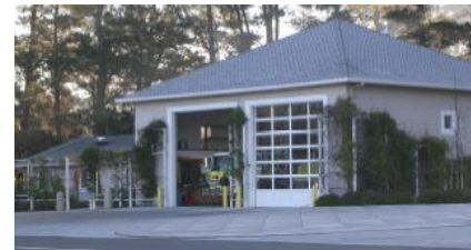
Station 74, completed in August 2002
