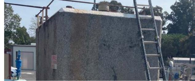
**Description:** In-kind replacement of a 4,000 gallon diesel storage tank used to supply fuel to standby generators and City vehicles. The existing tank is compromised.
