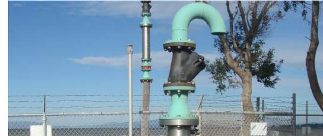
**Description:** Effluent pumping capacity of the treatment plant is limited by the capacity of the pipe size at the effluent outfall in Rodeo. Increasing the pipe size at the Effluent Outfall Eductor Station will increase the wet weather effluent pumping capacity and increase the lifespan of the effluent pipe by reducing the pressure in the line during storm events. Project requires coordination with Rodeo.
