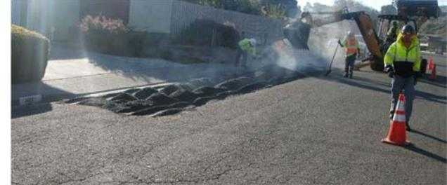
**Description:** Based on the most current P-TAP report various segments will be recommended for slurry seal treatment. A slurry seal functions as a topcoat to existing asphalt pavement to preserve and protect the pavement. It is best suited for pavements with mild to moderate damage, such as narrow cracks, but not for severe damage such as potholes.
