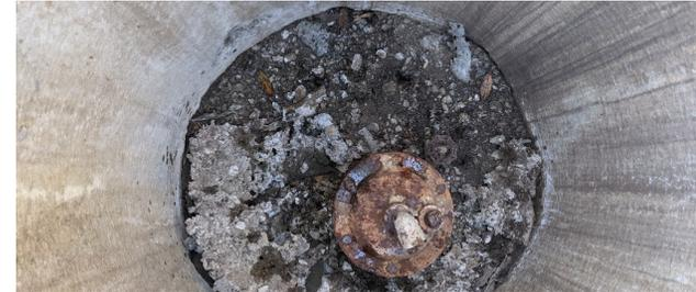
**Description:** There are four air relief valves at various locations on the WPCP Effluent Pipeline between the WPCP and the Rodeo treated water discharge point. This project includes removal and replacement of the pipe saddle, short pipe section, isolation valve, and air relief valve.
